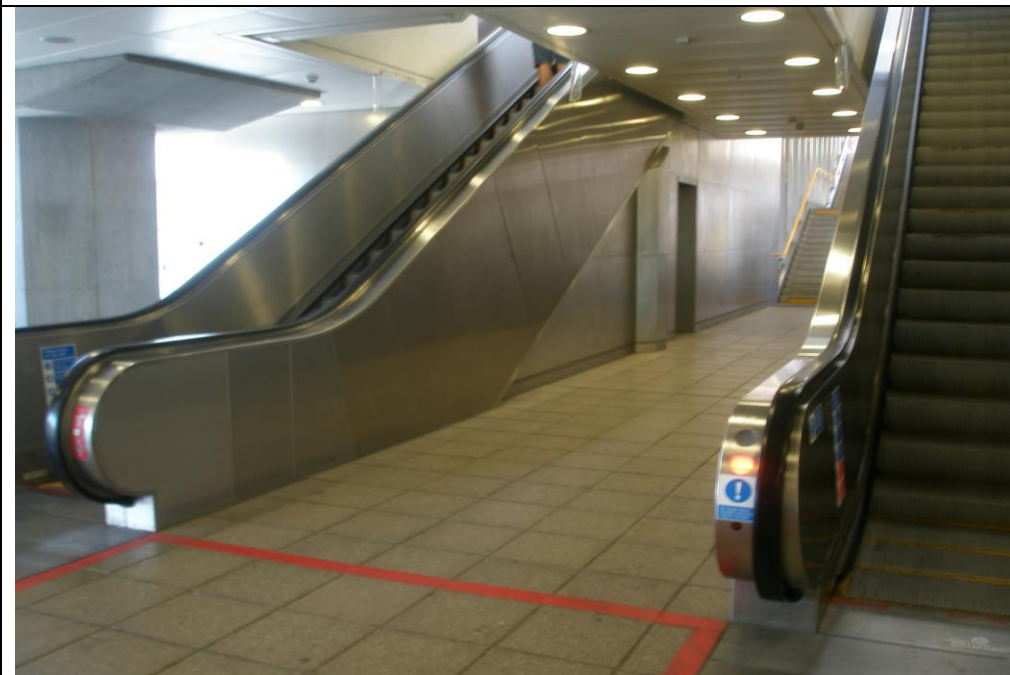
Escalator 2 Ticket Hall Level
