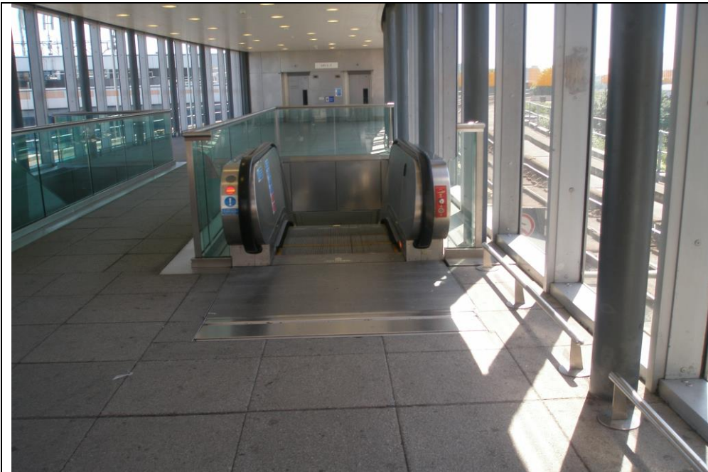
Escalator 2 Platform Level
